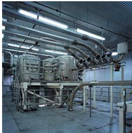
Vacuum weighing system for mixer with manifold valve.
