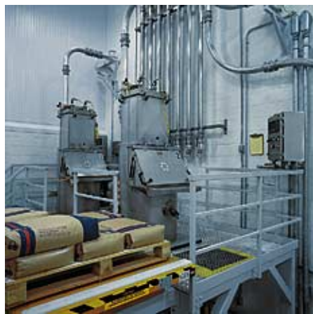
Bag tipping into the closed system.
